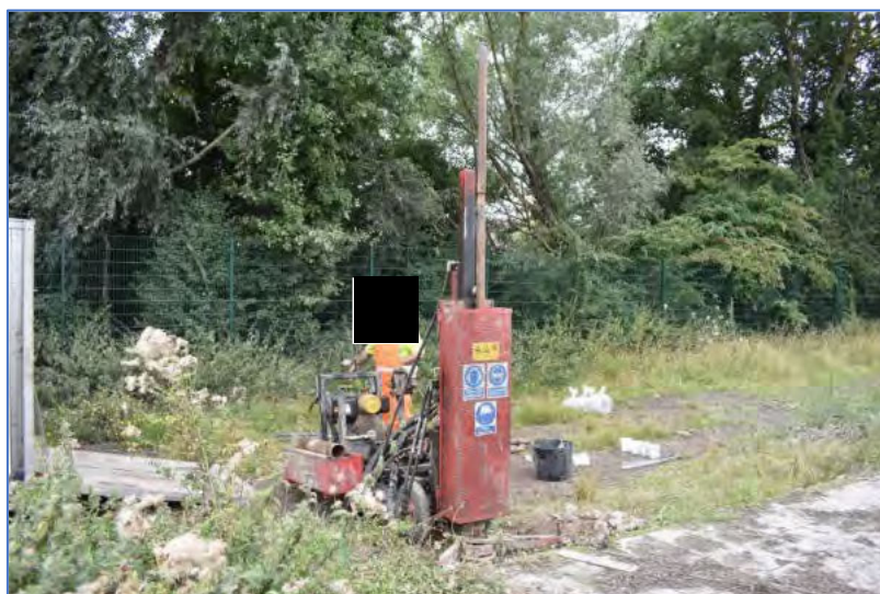
Plate 1: Dart 2 rig working shot from south
